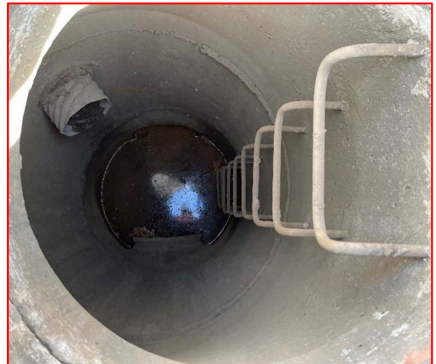
Photo 4 - Interior of Manhole
