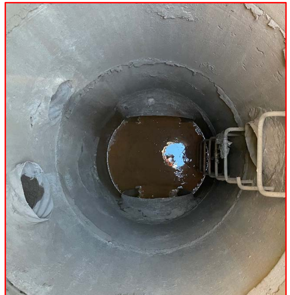
Photo 4 - Interior of Manhole
