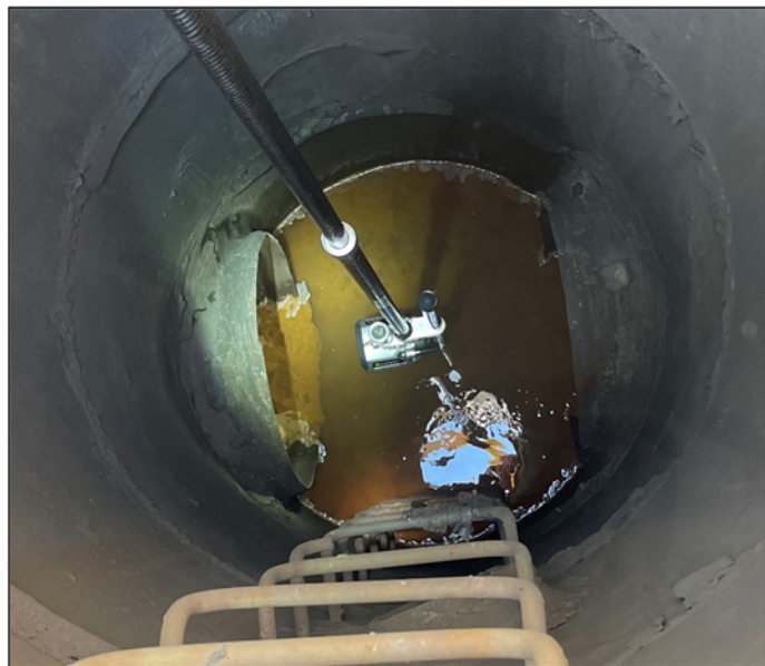
Photo 1 - Quickview Camera in Manhole 039
