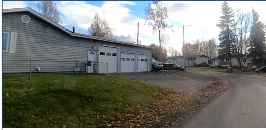
Parcel 20 (west) driveway has no landing, the driveway grade is over the DCM maximum, the driveway is wider than allowable, and the garage is located only 8' from the property line which requires parked vehicles to park in the ROW
