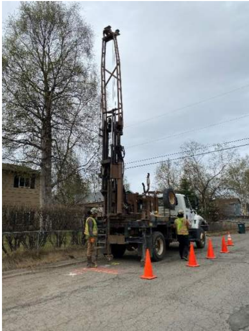
05/11/2021: Setting up rig on BH-01 with utility markings (left). Borehole marked with white paint. BH-01 after completion as a piezometer with flush-mount monument (right).
