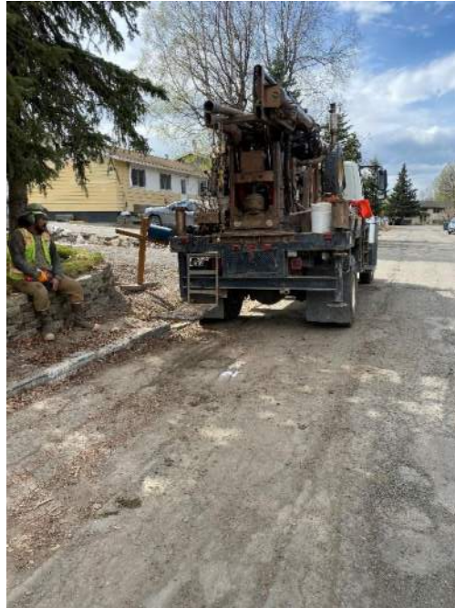
05/11/2021: BH-02 after completion of drilling and cold patch (no piezometer).
