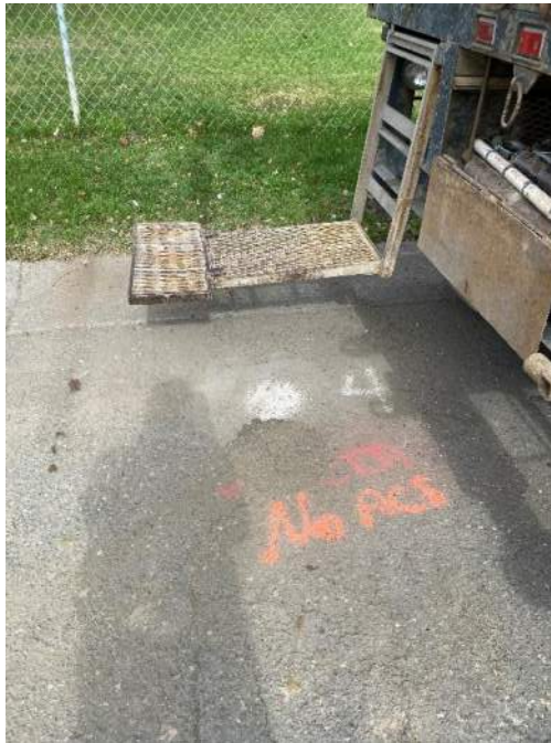
05/11/2021: BH-04 after drilling and completion. Backfilled and cold patched.
