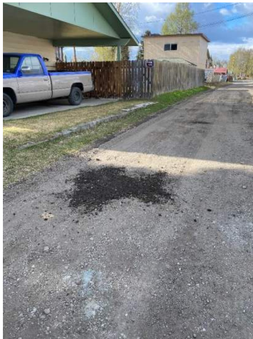
05/11/2021: BH-06 after completion. Hole was backfilled with cuttings from this hole and gravel was spread at surface and leveled.
